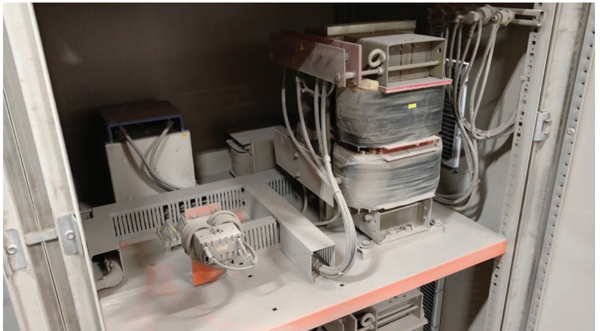
Dirty, overheated power supplies
